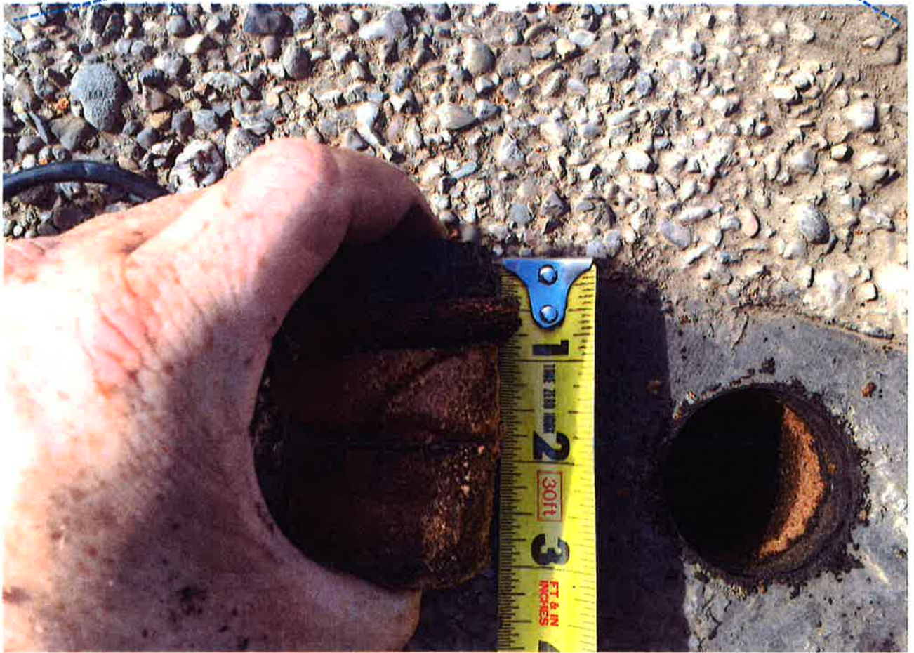
View of Test Core # 2
