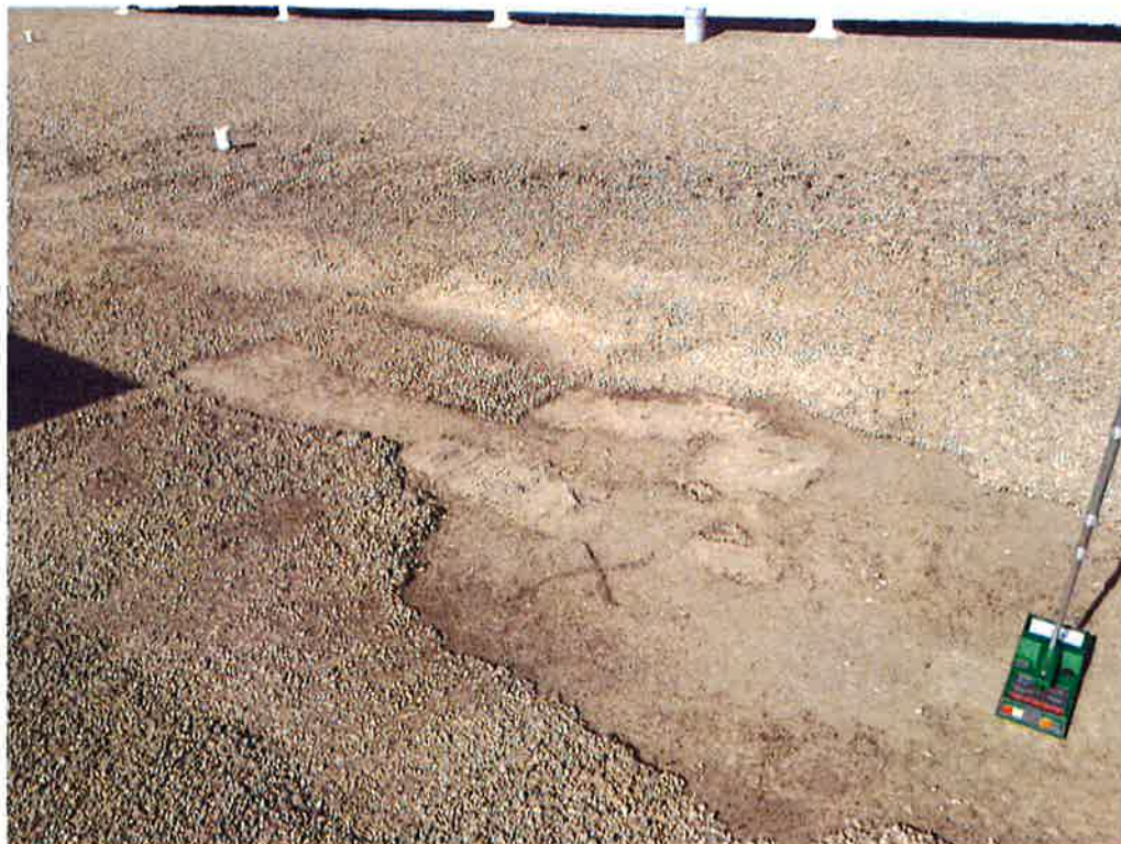
View of Test Core # 1 Area
