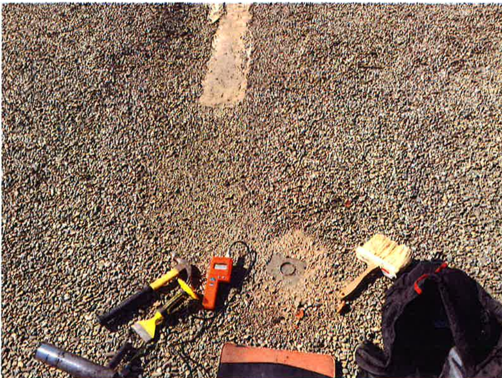
View of Test Core # 2 Area
