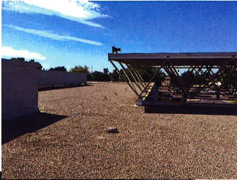
General view of roof
