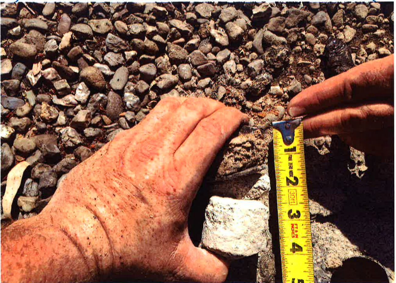
View of Test Core #3
